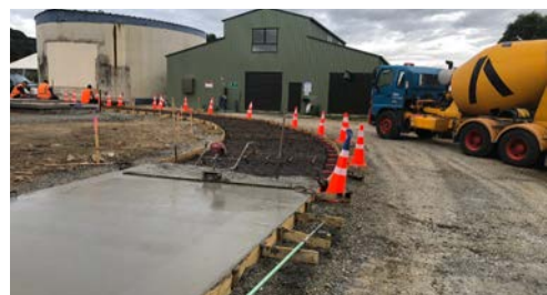
NEW DRIVEWAY TO SITE
