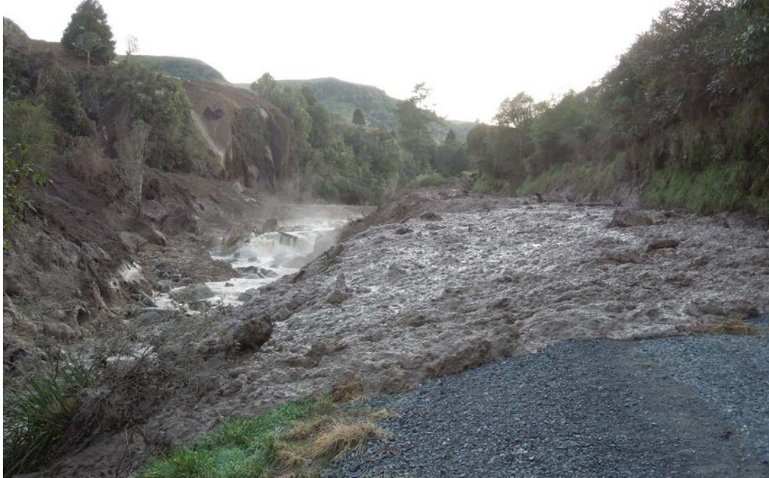
MUD AND DEBRIS AS A RESULT OF SLIP ON MANGANUI ROAD
