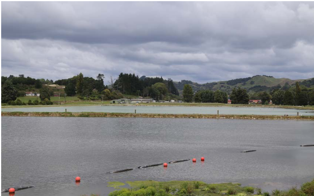
PONDS AT TE KUITI WASTEWATER TREATMENT PLANT
