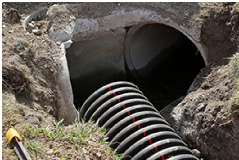
UPGRADE OF STORMWATER DRAIN EDWARD STREET
